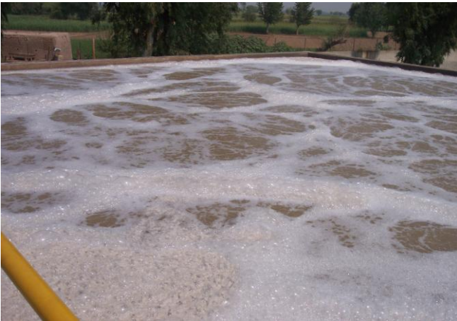
Fig. 5 Filled Aeration tank
