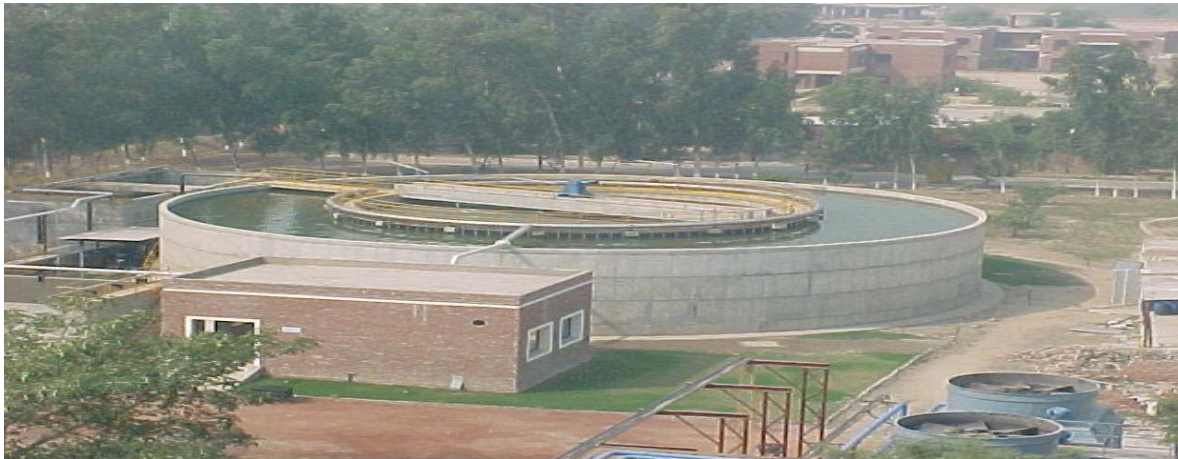
Fig. 6 Compact Treatment Plant at ICI, (Capacity 25.92 M 3 /Hr.) CTP UNIT [8]
